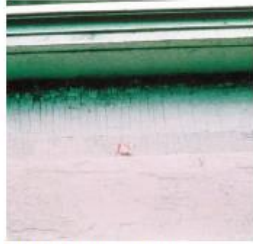
FIGURE 5.4b Alligatoring paint
