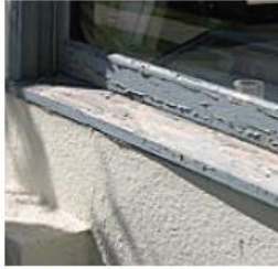
FIGURE 5.4a Peeling paint
